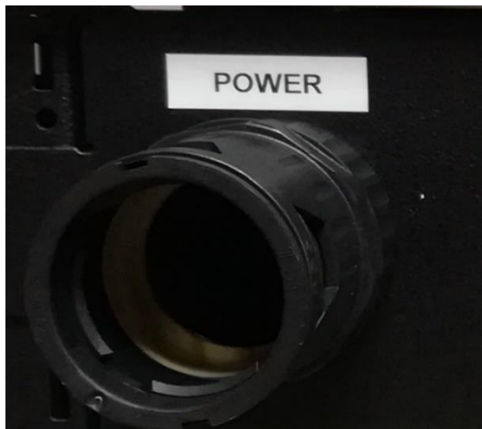
Figure 6: Power supply bulkhead union
